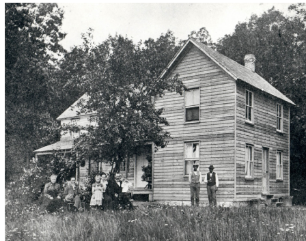
Otis Mason House, c. 1900, a National Trust for Historic Preservation property, located at former Woodlawn Stables, was moved recently for Route 1 widening work.
